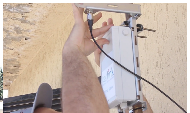
Libatel team installing Kerlink's LoRaWAN™ Wirnet™ Station
