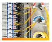
The patch cord management colour system enables you to install, locate and trace individual fibres along easy-to-follow cable routing paths.
